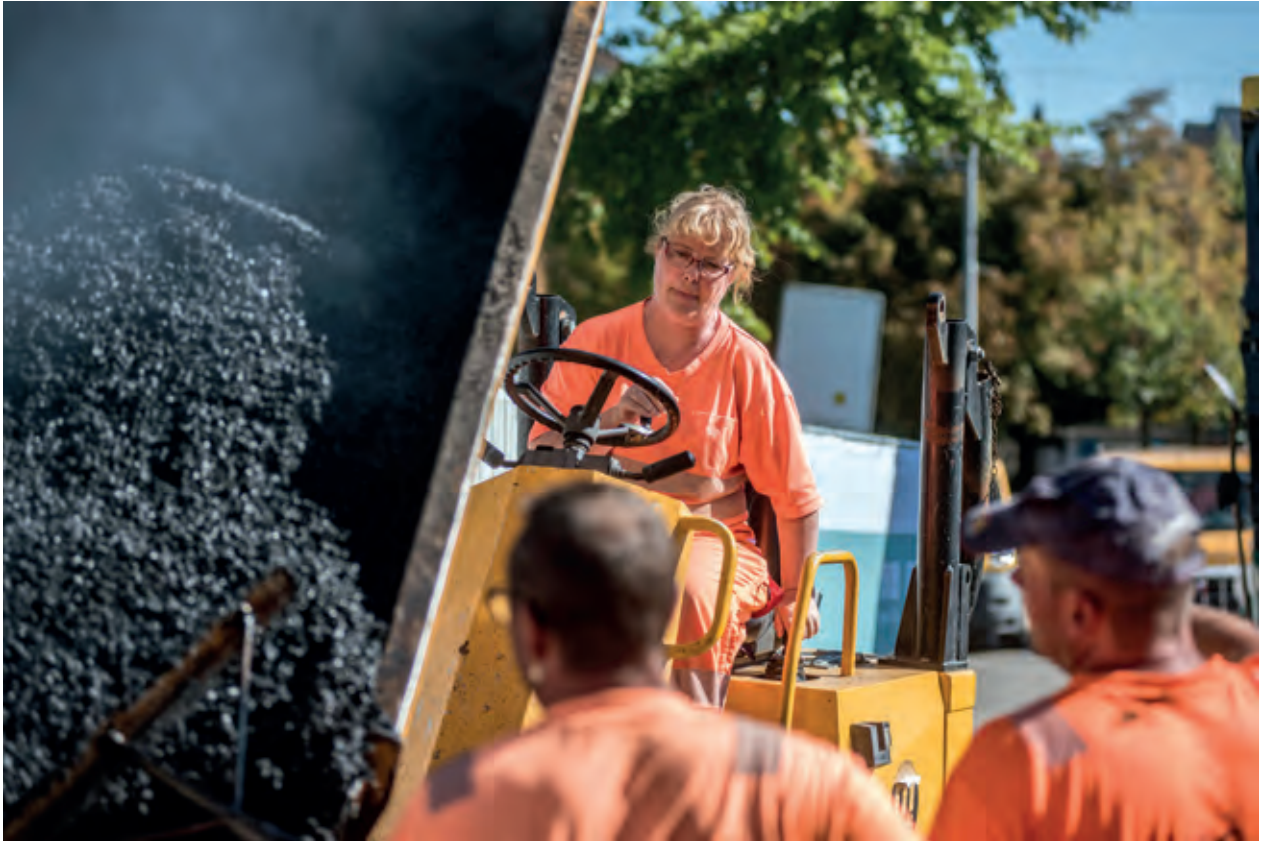
Photo series "Sanierung Kirchenfeldbrücke", 2018 © Alexander Egger"
