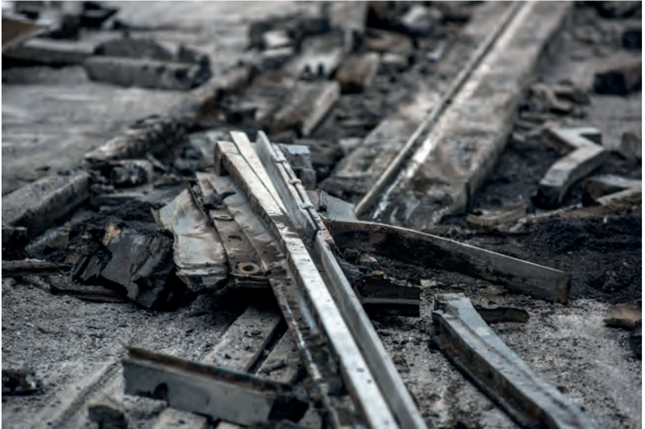
Photo series "Sanierung Kirchenfeldbrücke", 2018 © Alexander Egger"
