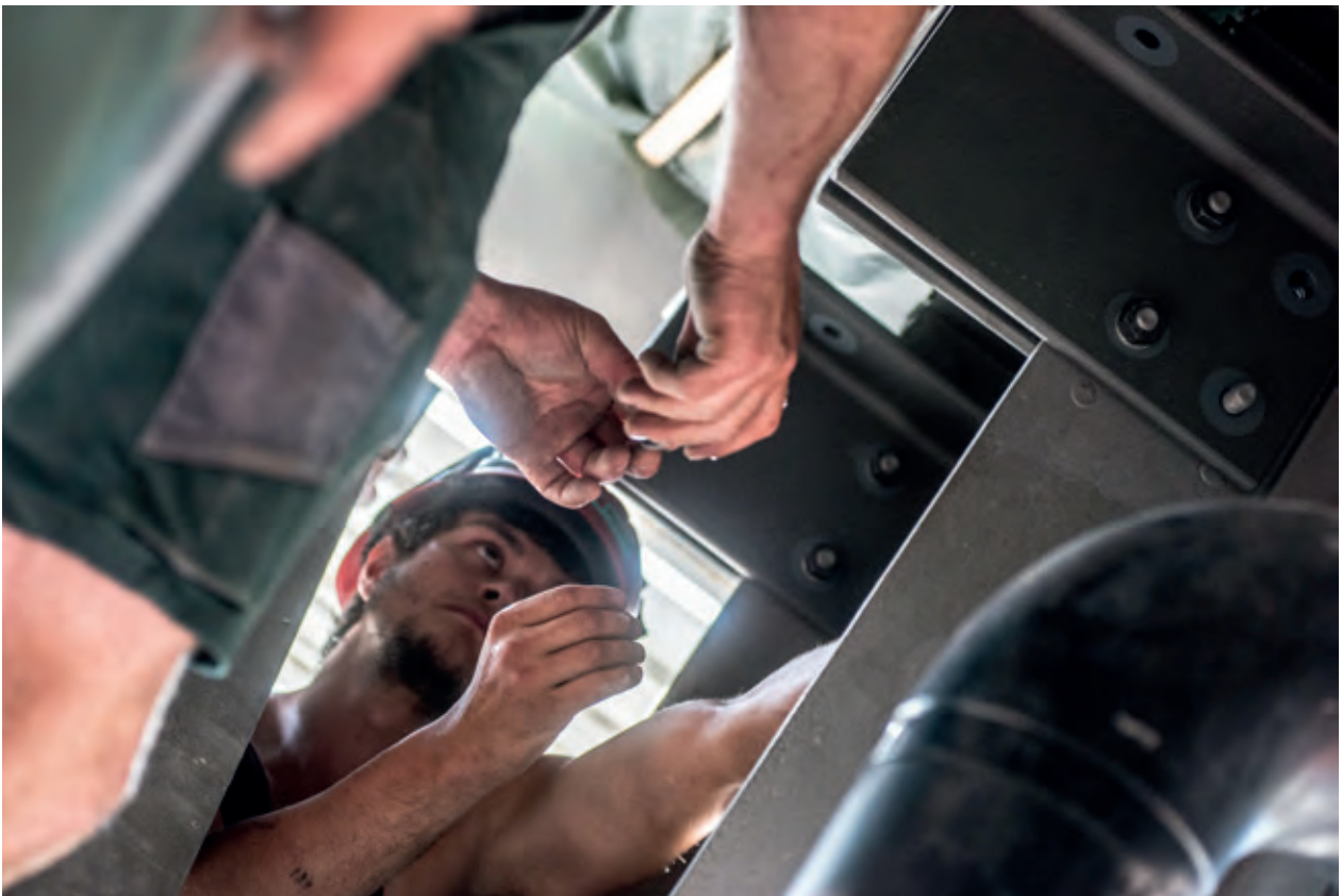
Photo series "Sanierung Kirchenfeldbrücke", 2018 © Alexander Egger"
