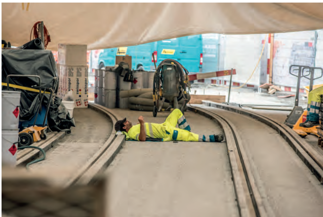
Photo series "Sanierung Kirchenfeldbrücke", 2018 © Alexander Egger"
