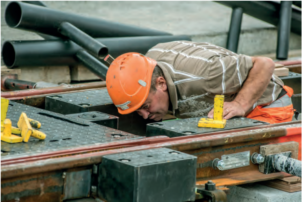
Photo series "Sanierung Kirchenfeldbrücke", 2018 © Alexander Egger"
