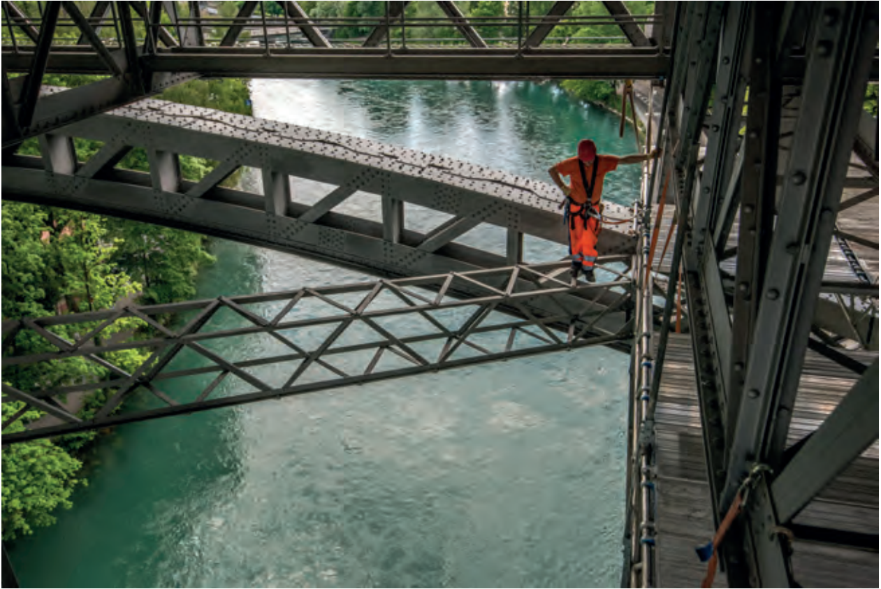
Photo series "Sanierung Kirchenfeldbrücke", 2018 © Alexander Egger"
