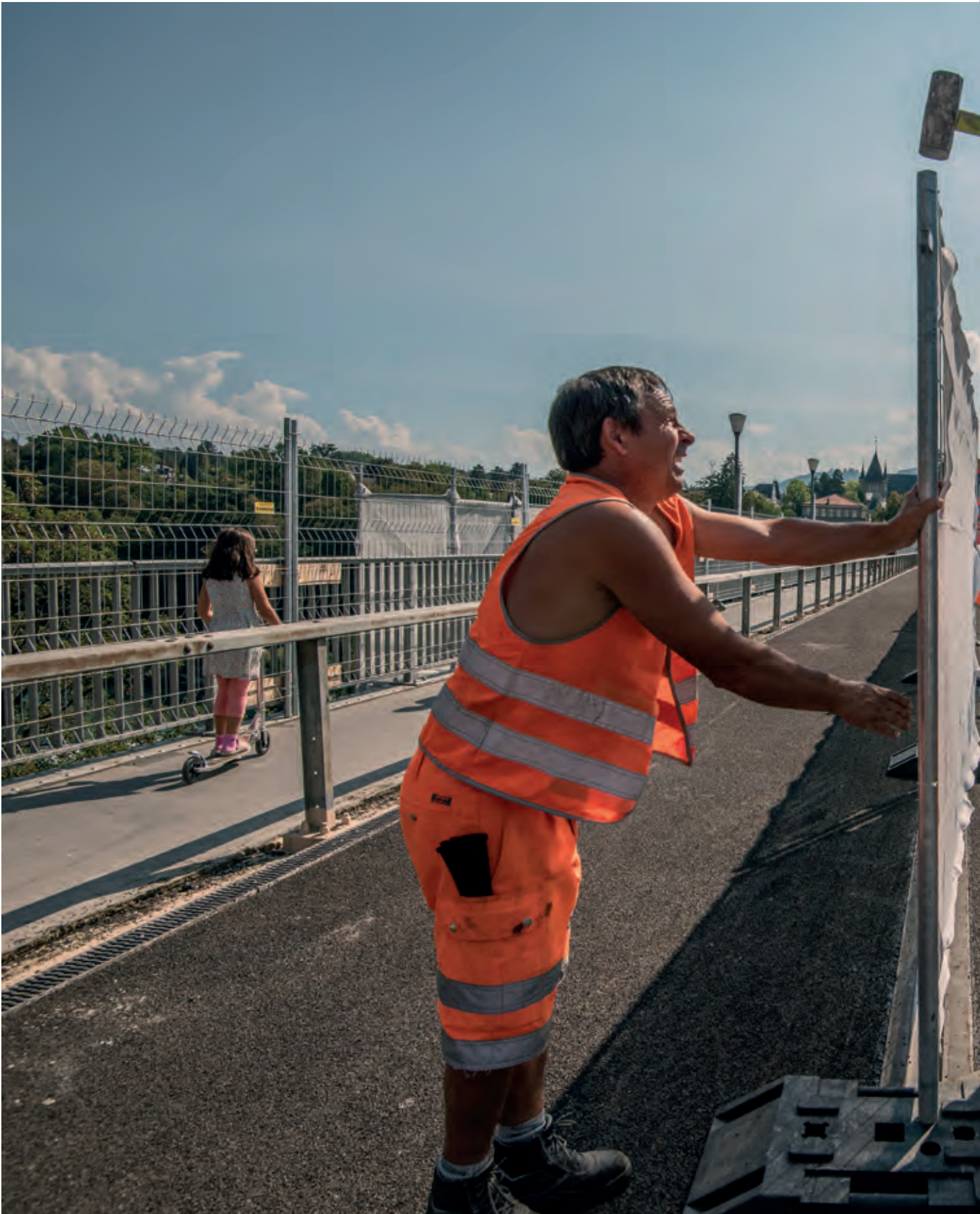
Photo series "Sanierung Kirchenfeldbrücke", 2018 © Alexander Egger"
