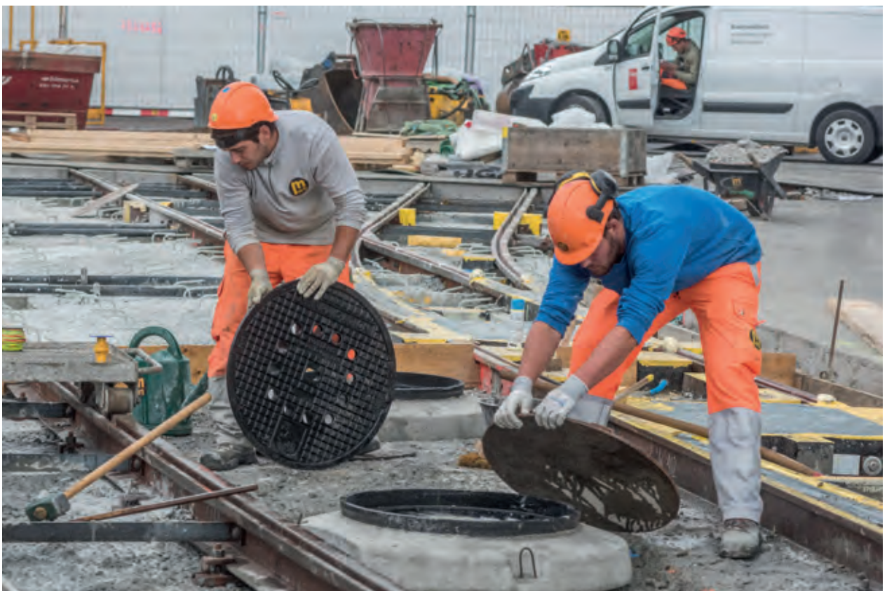
Photo series "Sanierung Kirchenfeldbrücke", 2018 © Alexander Egger"
