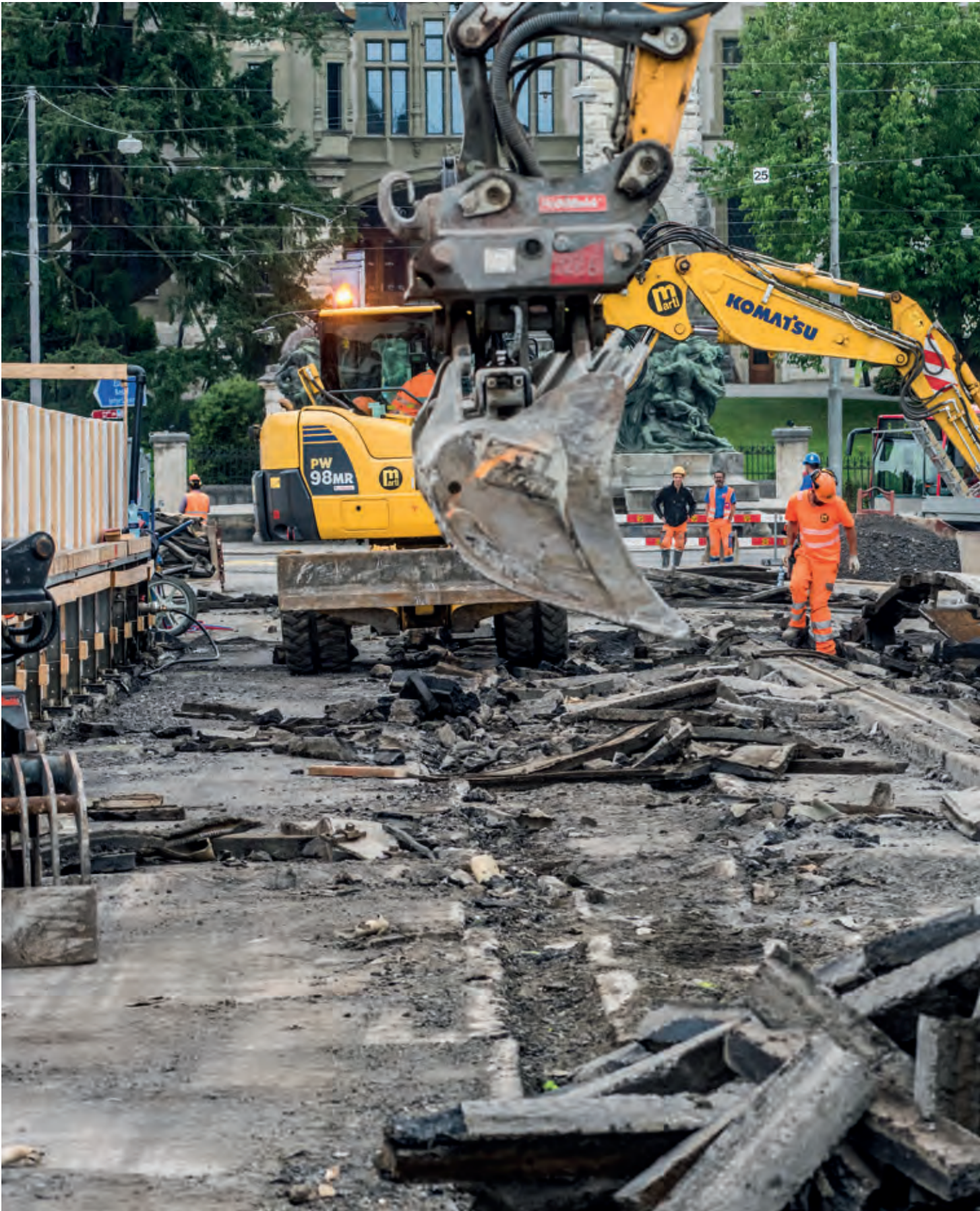
Photo series "Sanierung Kirchenfeldbrücke", 2018 © Alexander Egger
