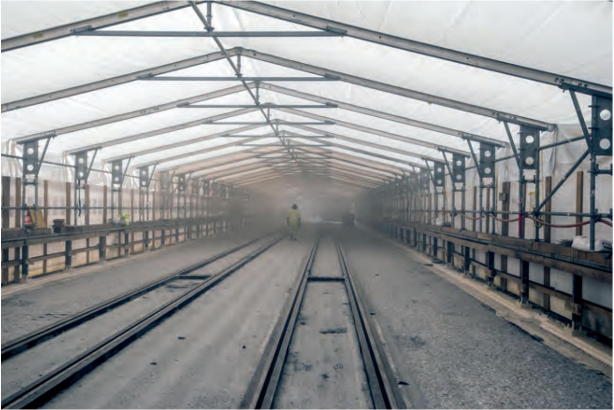
Photo series "Sanierung Kirchenfeldbrücke", 2018 © Alexander Egger"
