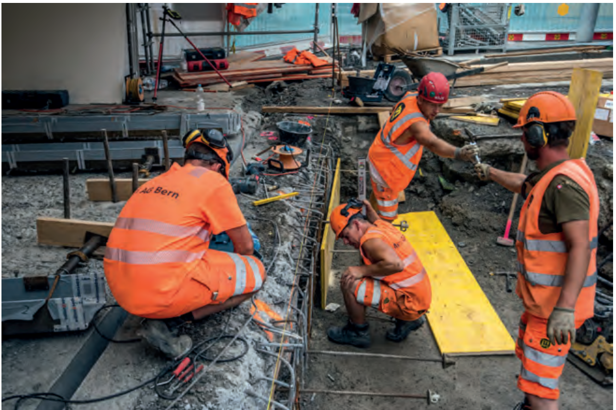
Photo series "Sanierung Kirchenfeldbrücke", 2018 © Alexander Egger"
