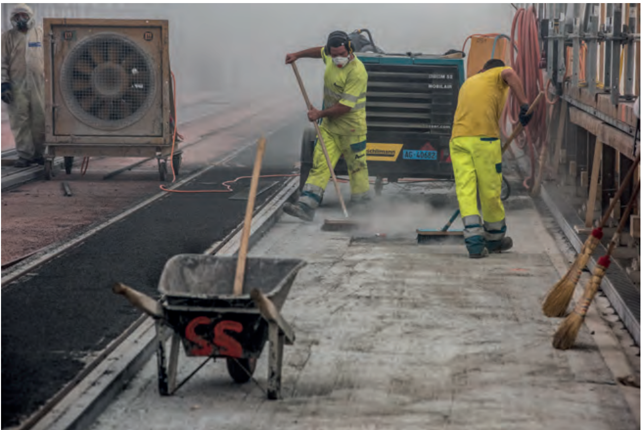
Photo series "Sanierung Kirchenfeldbrücke", 2018 © Alexander Egger"
